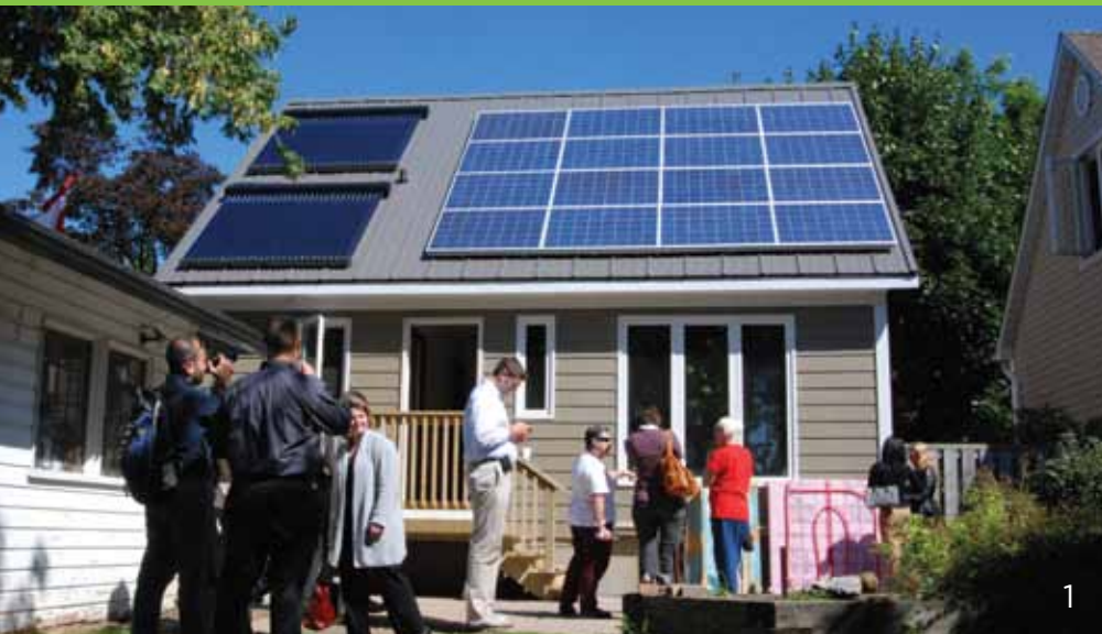
[1] THE FIRST NOW HOUSE RETROFIT IN TORONTO USED A SOLAR THERMAL SYSTEM FOR HEAT AND HOT WATER AND GRID-TIED SOLAR PHOTOVOLTAIC PANELS TO PRODUCE ELECTRICITY. WITH ONTARIO'S FIT SOLAR REBATES, THE HOME ACHIEVES A NET-ZERO ENERGY COST AND NET INCOME OF APPROXIMATELY $1100 ANNUALLY. PHOTO BY: HEIDI NELSON.
